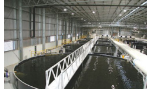
The design is focused on enabling a single operator to move fish from and to anywhere in the plant without having to net or handle them. Apart from the saving on labour, stress on the fish is minimized.
